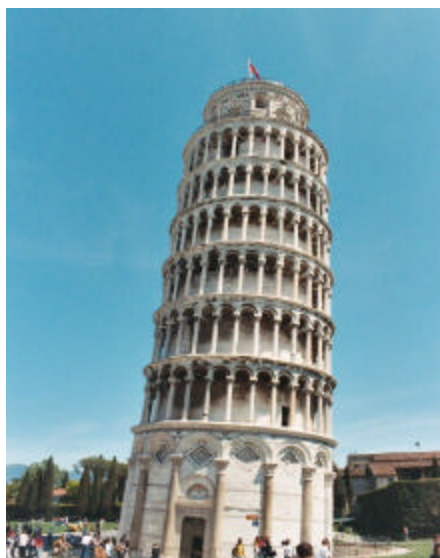
Leaning Tower of Pisa
